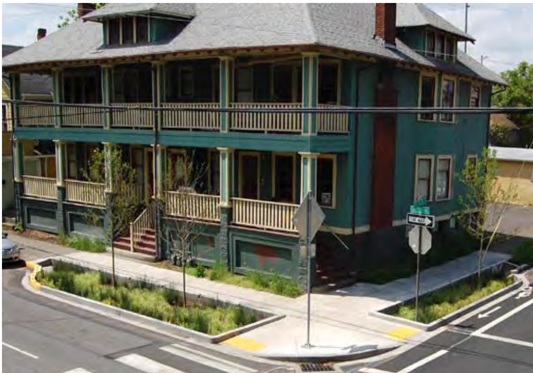
Curb extension with bioswales and street trees (Portland, OR).
