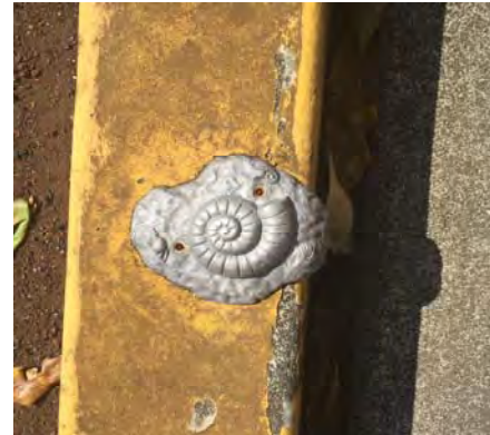
Hilo’s County Building and sidewalks feature decorative decals with ocean motif to discourage skateboarding use while adding a design element.
