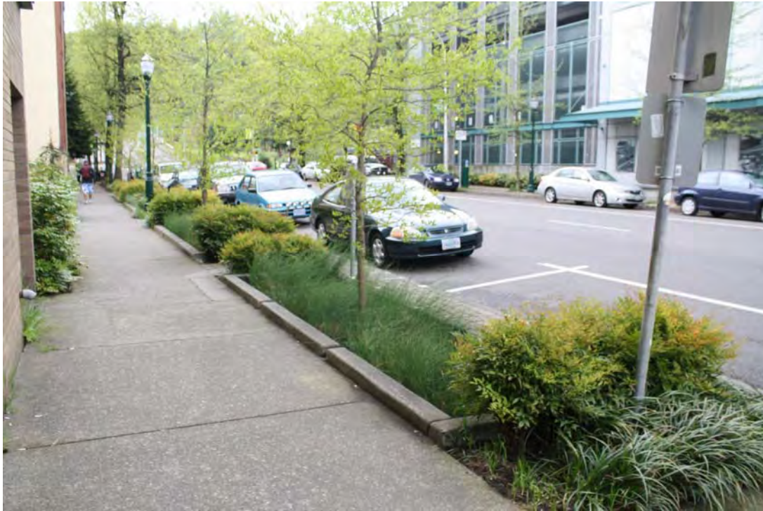
Example of an urban Green Street design using a continuous bioswale planter with drain inlets along the sidewalk and parking lane. (Portland, OR).
