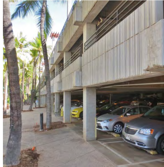
Parking garage at Fort DeRussy in Waikīkī.
