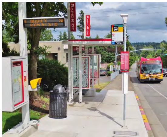
A bus stop in Bellevue, Washington on NE 8 th Street with real time schedule information, off board fare ticket vending machine, transit system map, route map and schedule and extensive branding.
