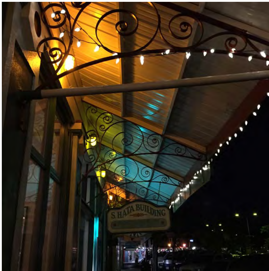
Illuminated awnings exist along storefronts lining Kamehameha Avenue Frontage Road
