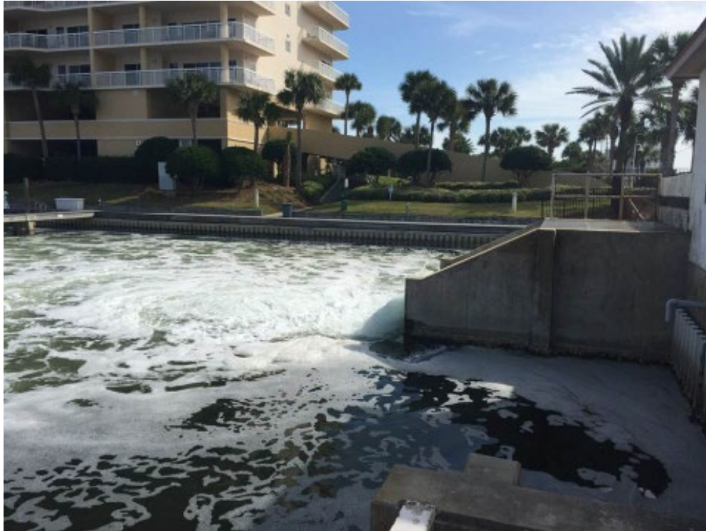
Figure 9 Destin Harbor Pump System with concrete enclosure, Florida (getthecoast.com)
